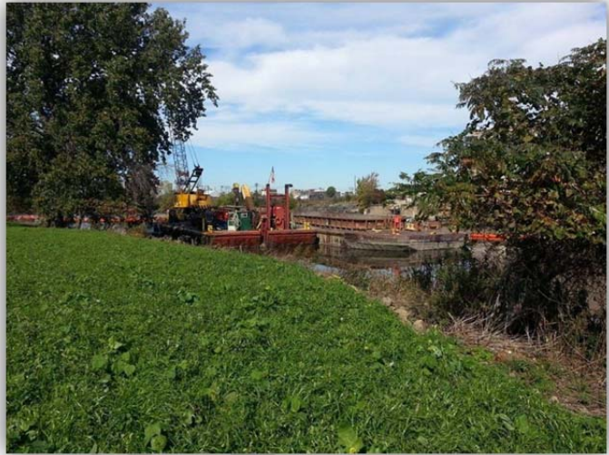
Phase II of Buffalo River Dredging (2013)
