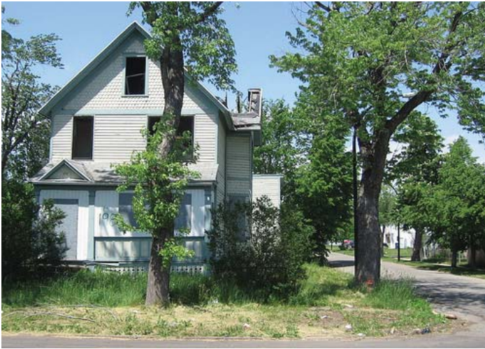
Vacant Home, City of Buffalo Source: Buffalo Niagara RIVERKEEPER
