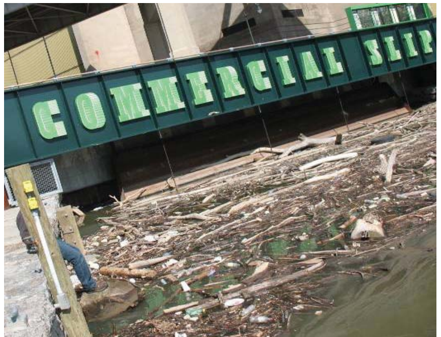
(Above) Commercial Slip Source: Buffalo Niagara RIVERKEEPER
