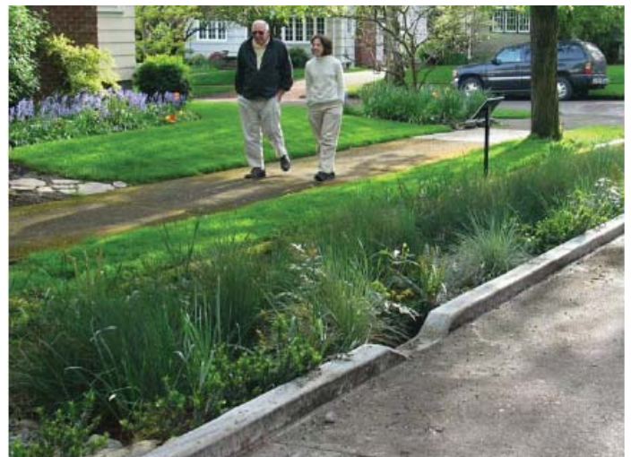
Bioretention area alongside traditional tree lawn.
