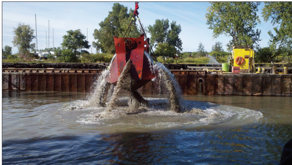
A dredge bucket is raised from the City Ship Canal in the first phase of dredging, September 2011.
