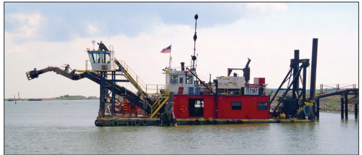
U.S. Army Corps of Engineers barge loader, “Lucille T.,” which transfers dredged sediment to the Confined Disposal Facility
