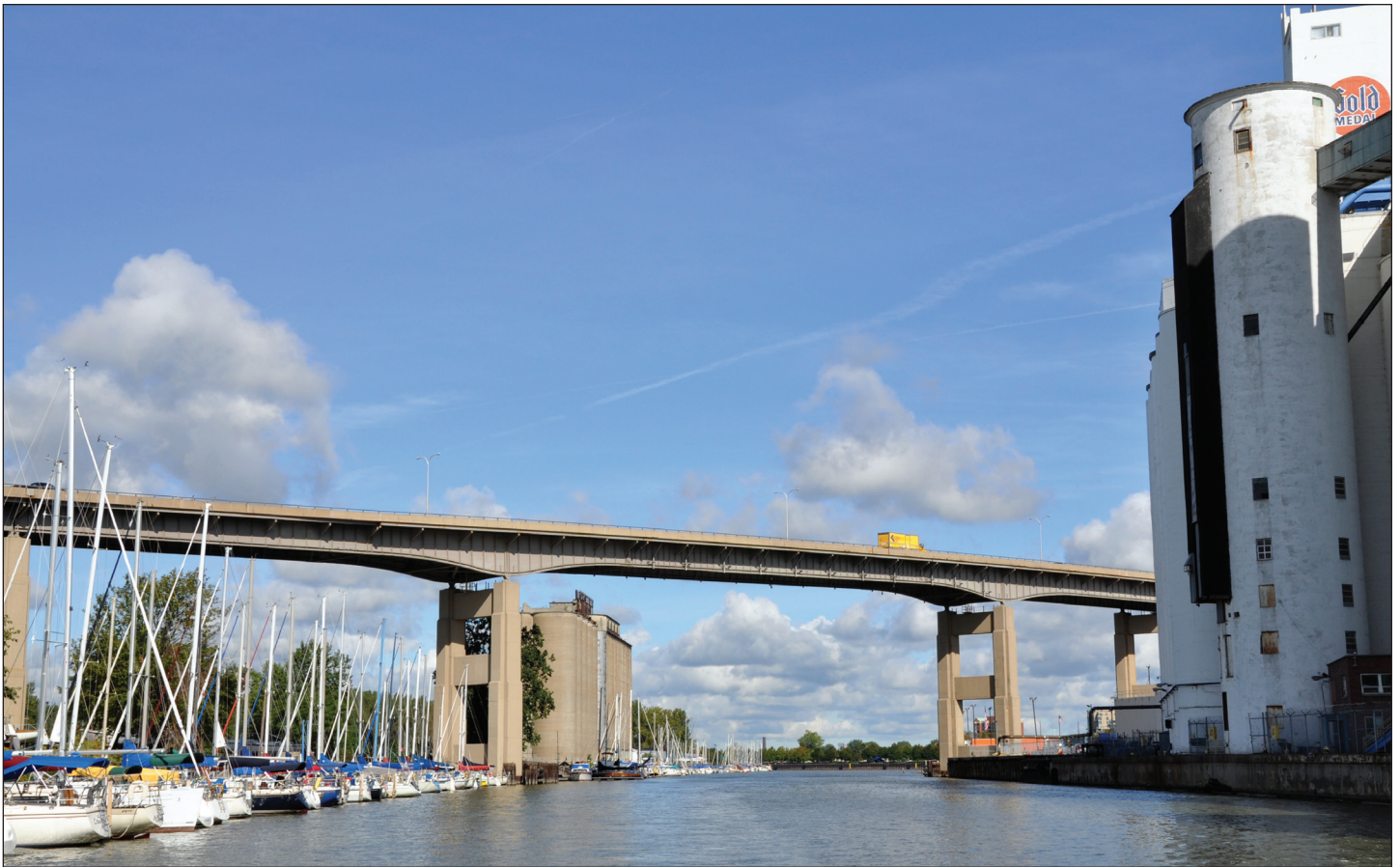
Looking at the Skyway Bridge from City Ship Canal
