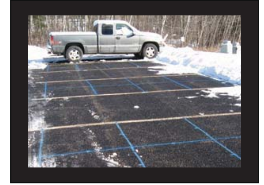
Pervious Pavement in winter months help reduce slush and slick surfaces. (Photo taken 1 hour after plowing) No salt or sand was used, only infiltration from porous asphalt.
