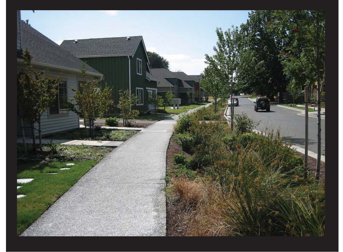
Above: (Green Infrastructure) This design was installed in Portland, Oregon. Shown on a dry weather day. The stormwater helps to irrigate the garden as well as reducing the amount of stormwater entering the sewer system.
