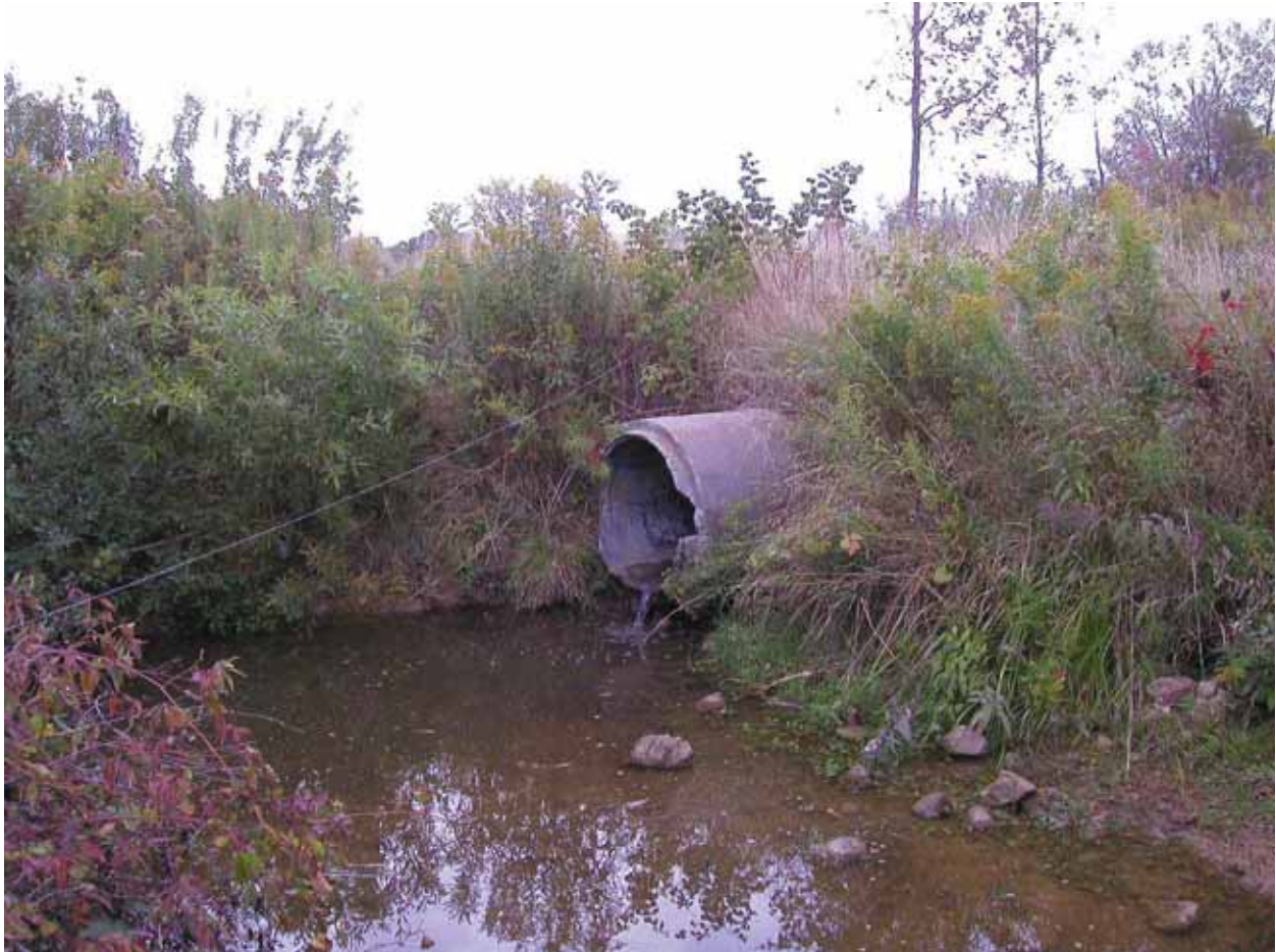
FIGURE 2.5.3-24 HANGING CULVERT ON REACH CET1
