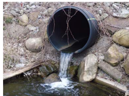
Perched culvert that presents impassible conditions due to height and low flow (BNR).
