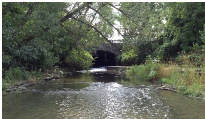
The Scajaquada Drain in Forest Lawn Cemetery- the point at which Scajaquada sees daylight after traveling underground for 3.7 miles.
