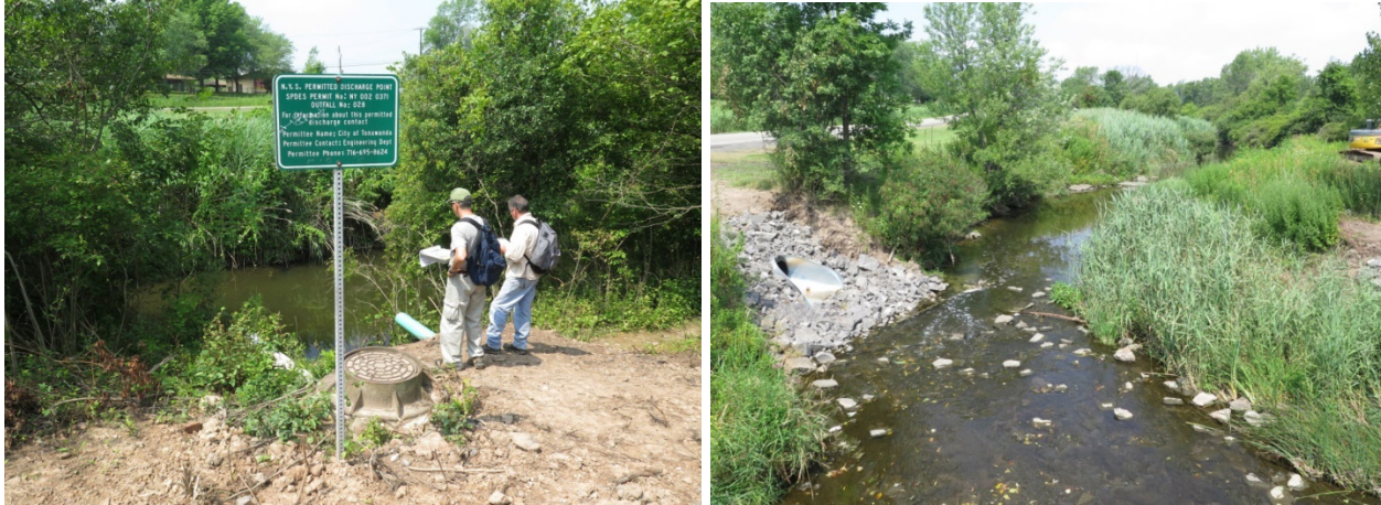
Left: Permitted discharge location along Two Mile Creek downstream of the Fletcher Street Bridge. A need for erosion and sediment controls were observed at this location. Recommendations include mulching, seeding, and plantings to address soil erosion and to restore riparian structure. The installation of a rock splash apron for the discharge and in-stream structure would also enhance fish habitat. Right: A view of Two Mile Creek looking upstream from Fletcher Street Bridge. A lack of overhanging vegetation and disturbance due to drainage associated with construction is evident.
