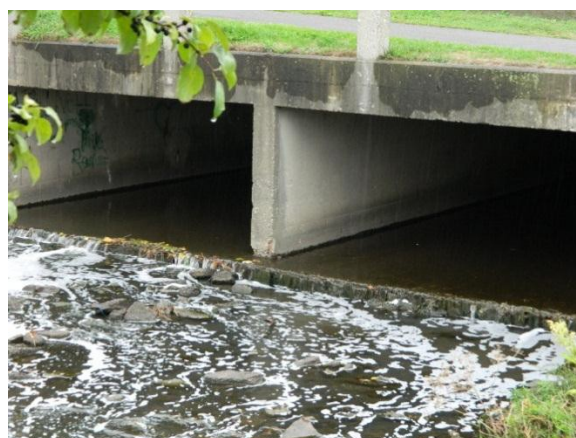
This box culvert along Two Mile Creek includes an approximately six inch ledge that presents impassible conditions for warmwater fish species.
