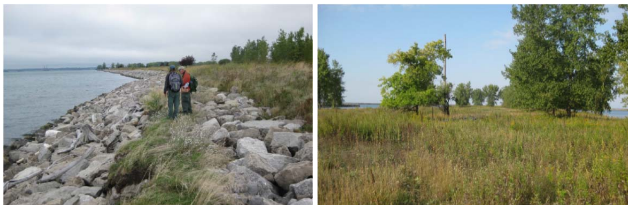
Left: Isolated sod deposit on riprap shoreline along Greenway Nature Trail. This area provides an existing example for naturalizing the shoreline using soil and robust native plants with strong and extensive root systems. Right: Peninsula between the Seaway Piers. This isolated site could be enhanced and managed as a wild area with limited recreational access to increase Lake Erie shoreline habitat values.
