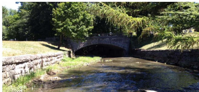
A channelized section of the creek within Forest Lawn Cemetery. The stream has narrowed naturally within the artificial walls.
