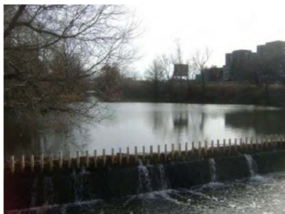
Finger dam that impedes fish passage to upstream areas of Scajaquada Creek.
