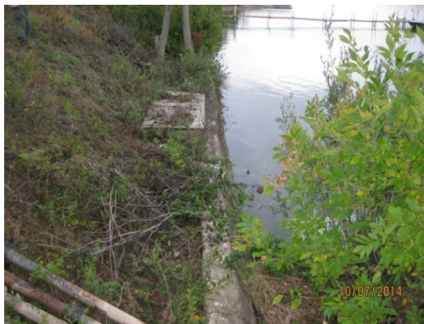
Left: Undermined bank and fallen trees along southern shore of Beaver Island State Park (Site 82). Right: Concrete wall at Site 84, facing south. The wall supports the steep bank; removal would likely cause bank failure.
