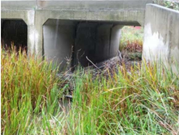
Left: First barrier along Bergholtz Creek. The culvert is in good condition however the site is heavily vegetated with Phragmites. Addressing vegetation and installing step pools will allow passage for minnow and panfish species. Right: Second barrier along Sawyer Creek. Vegetation removal would help achieve passage for minnow species to the upper reaches of the stream.
