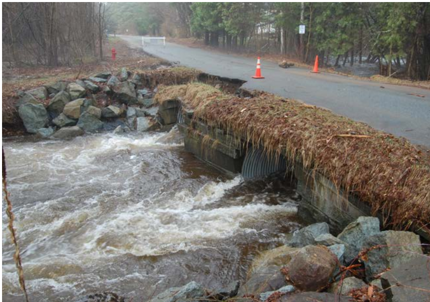
Figure 6: Original Culvert on Lewis Brook
