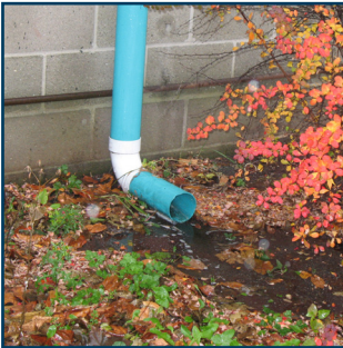
Downspout Disconnection
