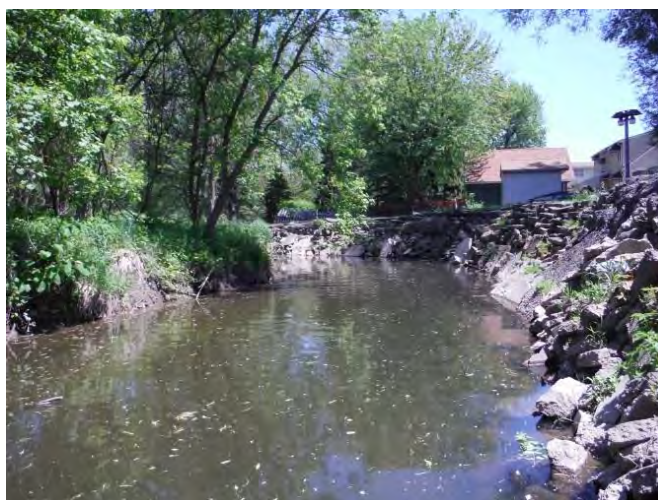
Figure 4.2: Altered Stream Channel with use of Rip-Rap (BNR)
