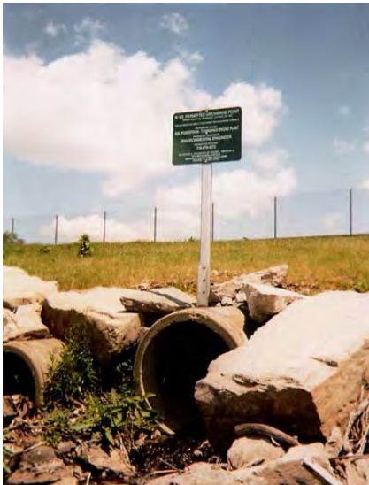
In our region, combined sewer outfall points are marked by a green sign.
