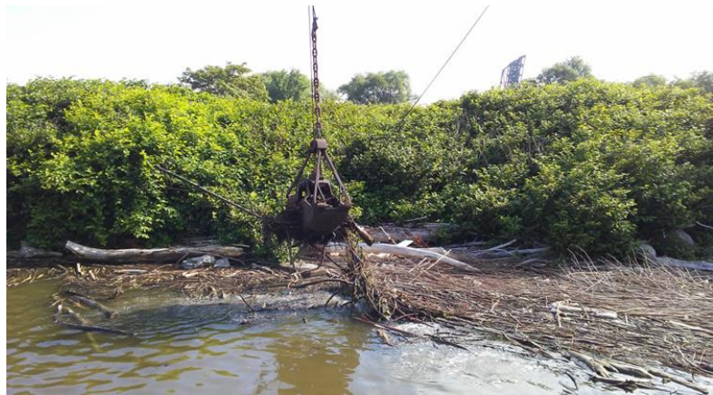
Figure 15. Three barges of large woody debris were removed from the “Blue Tower Turning Basin” site. The debris was removed from this site before in-water habitat was planted. A rootwad chain and floating boom system was then installed to deflect additional accumulation of debris.
