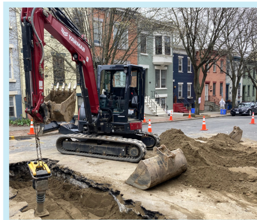
Photo 4: Lead pipe replacement in Albany.
