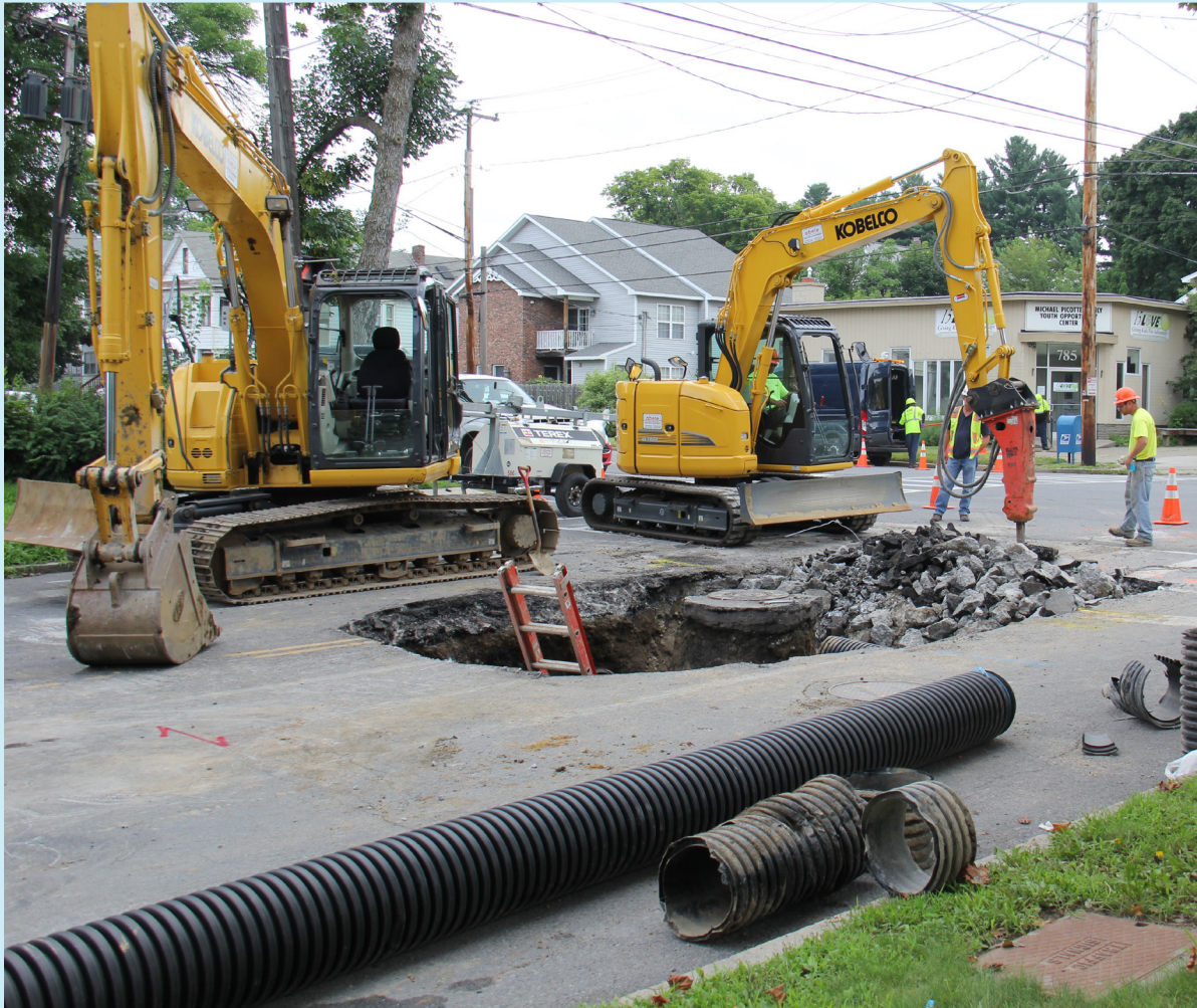
Photo 5: Water infrastructure upgradet in Albany.
