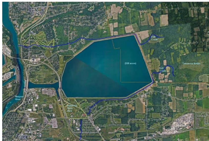
Figure 3. Aerial image of current NYPA Reservoir and Gill Creek with former boundary of Tuscarora Nation shown in a yellow outline. Source: Hidden Waters Blog.
