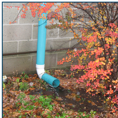
Downspout Disconnection
