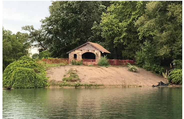
Pre-construction: Site conditions as of 2019
